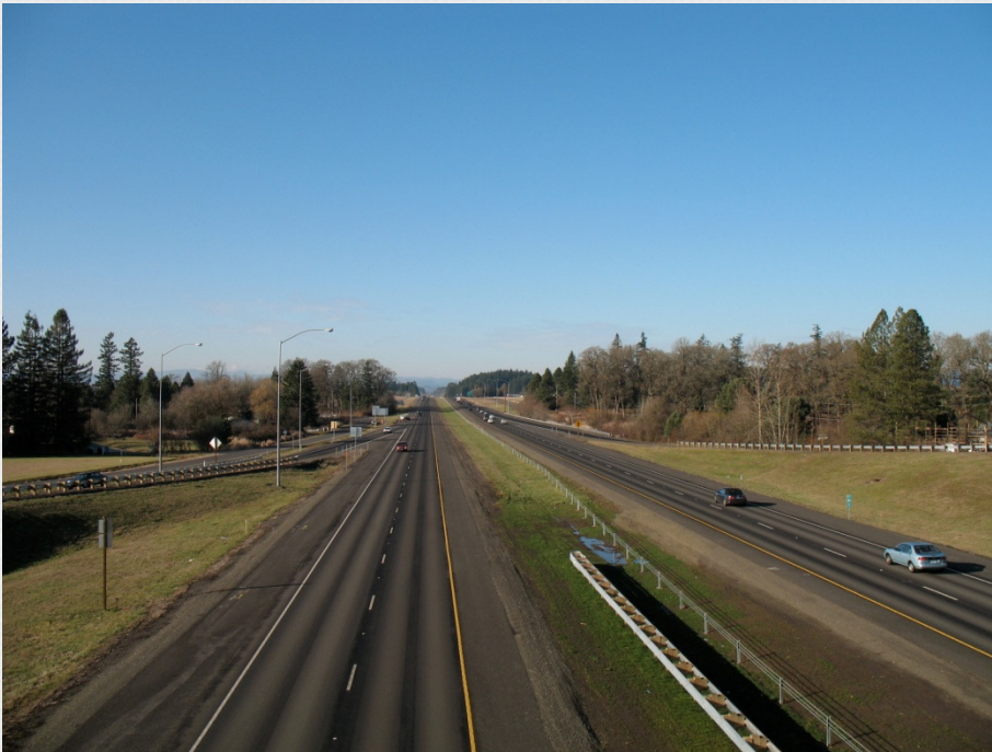
US-26 looking west from Helvetia Road overpass
